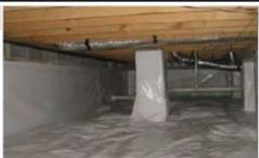
• Size of available vents should equal to 1.5% of the square footage within the crawl space. Relative humidity should be consistent with interior of home. Moisture content of sub floor should not vary more than a 2% MC from the top of the sub floor to the bottom.
